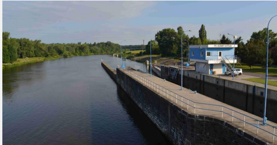
Water supply – Waterworks: Kalvary
