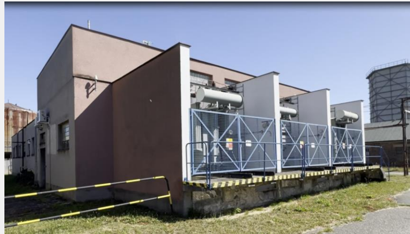
Energy building – Kolín production area
